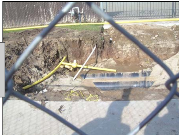
Underground Utilities at Ag. Entrance
